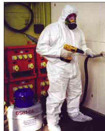
Using a Class H vacuum cleaner and a drill cowl
