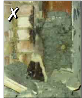
Broken asbestos insulating board, asbestos lagging and sprayed asbestos (limpet)
